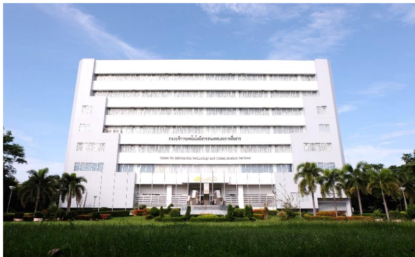
Figure 24 Center for Information Technology and Communication Services (CITCOMS) building
